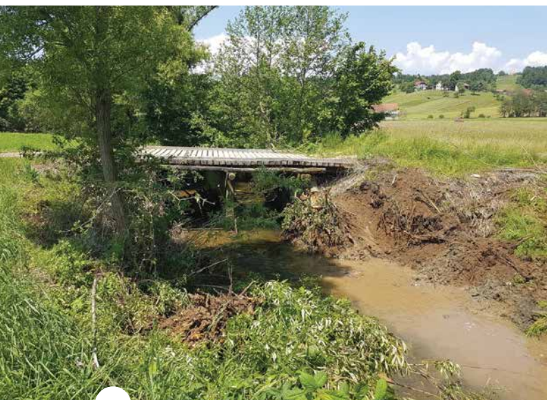
Most pred obnovo
